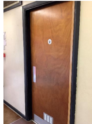
Girls' toilets by the hall
